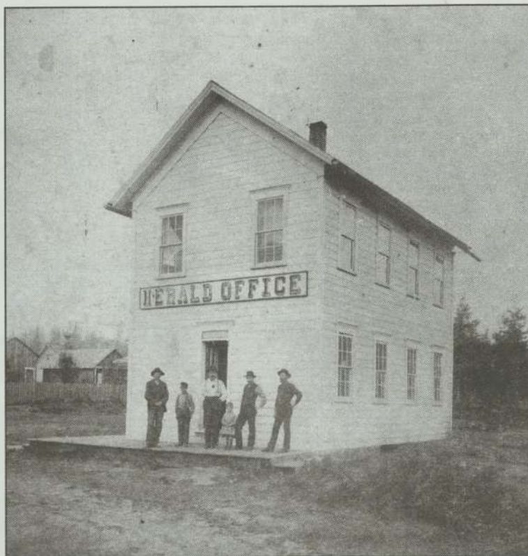
This building was likely The Coquille Herald's first home. Its location has been lost in the mists of time. This photo, and a 1883 issue of the newspaper, were graciously donated by Margaret Dean to The Sentinel this year .
