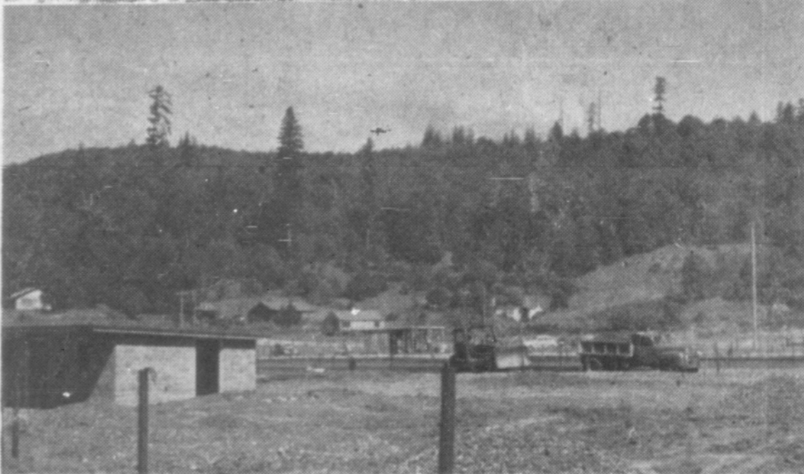
THEATRE AMONG THE FIRS —The Myrtle Lane Drive-In theatre is set in truly lovely surroundings up the Rink Creek road just a few blocks off the Myrtle Point-Coquille highway. Pictured above are some of the Sentinel photos taken during the last week of construction when all the workmen were busy preparing the grounds, setting the pipes, doing the wiring, and traveling, bulldozing, grading and completing the buildings. (Sentinel Photos)
