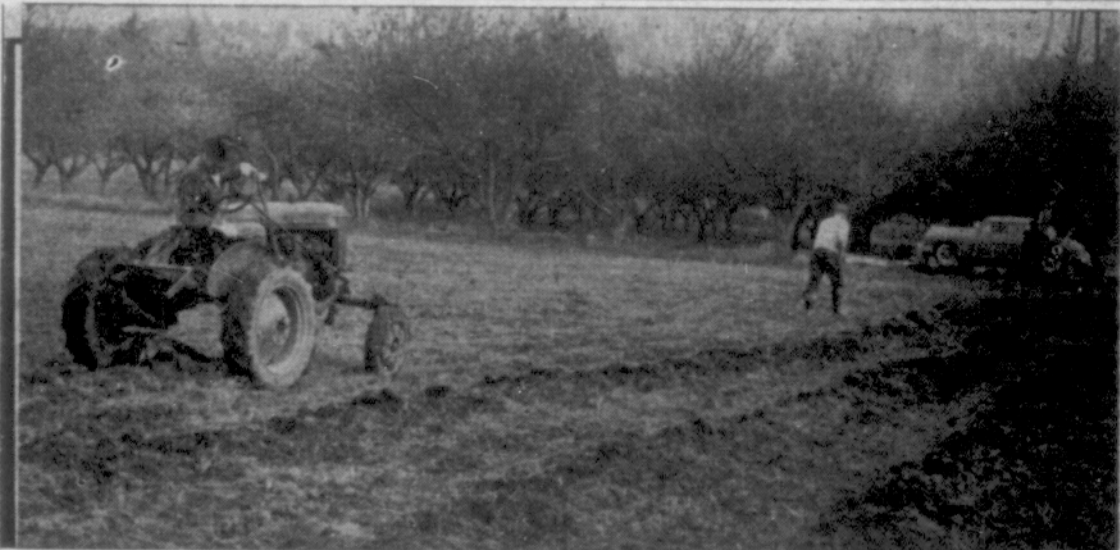
CONSTRUCTION scene shows Jess Dow helping to play out the ground wire for the new Radio KWRO. (Coquille Studio)
