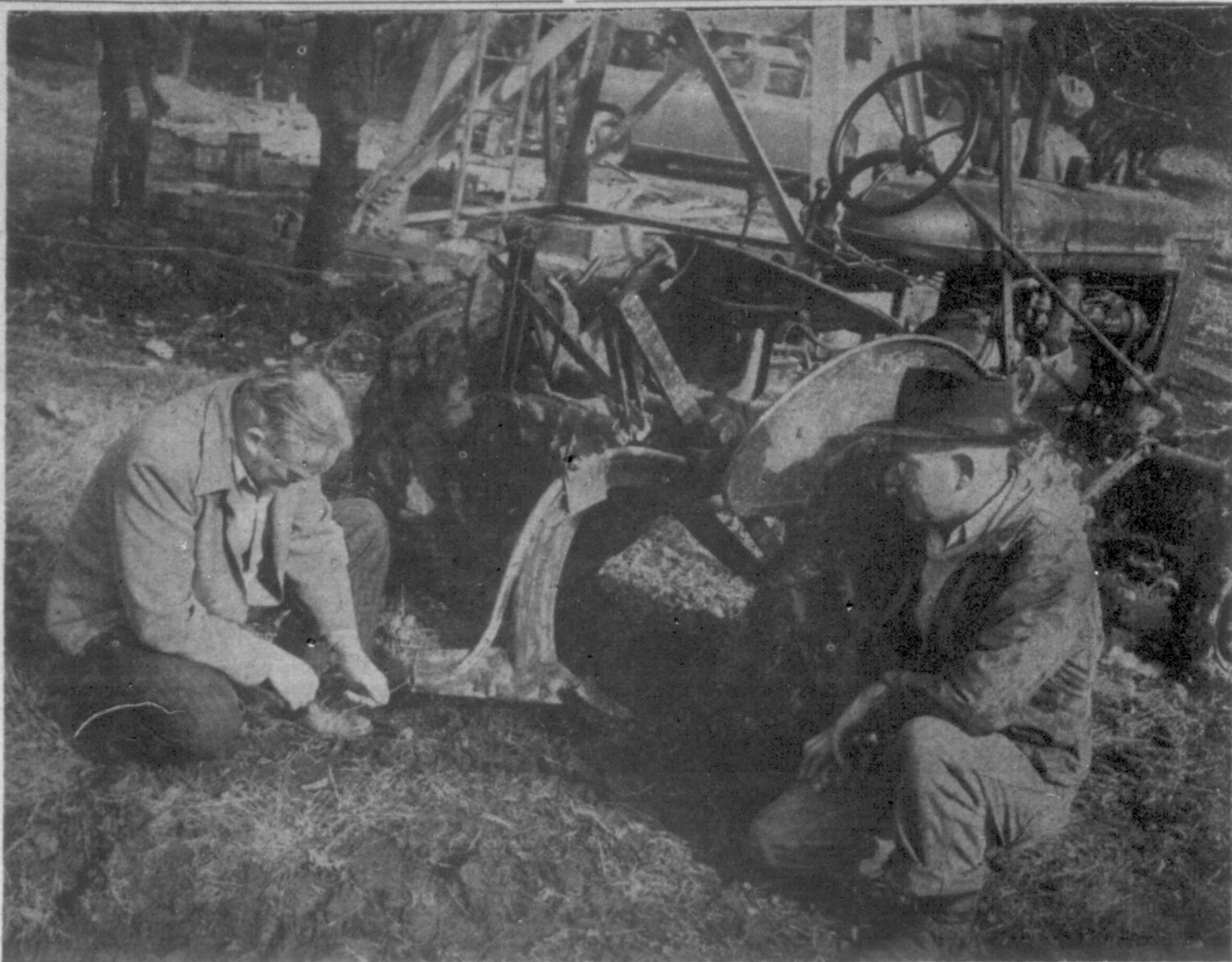
SOMETHING ENTIRELY NEW was developed when 22,000 feet of No. 8 bare copper ground wire was laid for the KWRO station. Pictured here are Walter Read, president, and E. W. Hall of Sanford Heights who worked out a special blade that placed the wire a foot or more in the ground in one operation.
