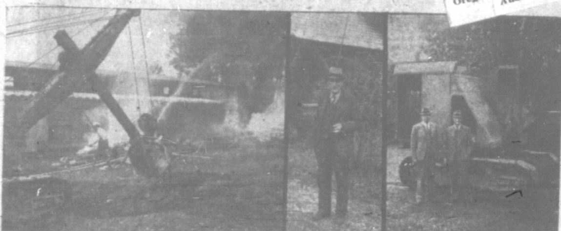
CHAIRMAN GEORGE ULETT AND MAYOR RALPH MILNE pose for a photo. Jack Lamb who was active in the project is snapped on the spot. Third photo shows some of the clean-up work in preparation of the site for the building. The Community building main committee was headed by George Ulett, chairman; Clarence Osika, secretary; and Bob Stewart, treasurer. This group served on the committee until the building was completed.
