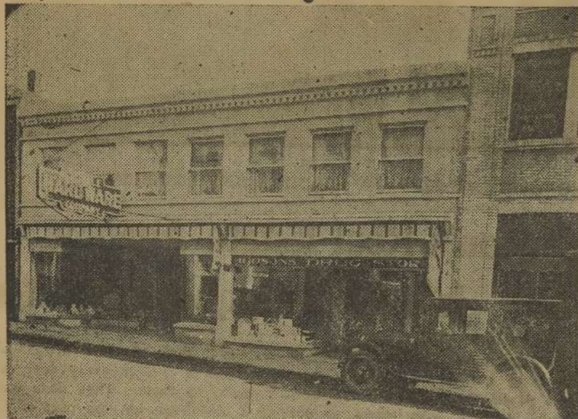
ELLINGSON BUILDING RECENTLY PURCHASED BY COQUILLE HARDWARE CO. OCCUPIED BY THEM AND HUDSON DRUG STORE
