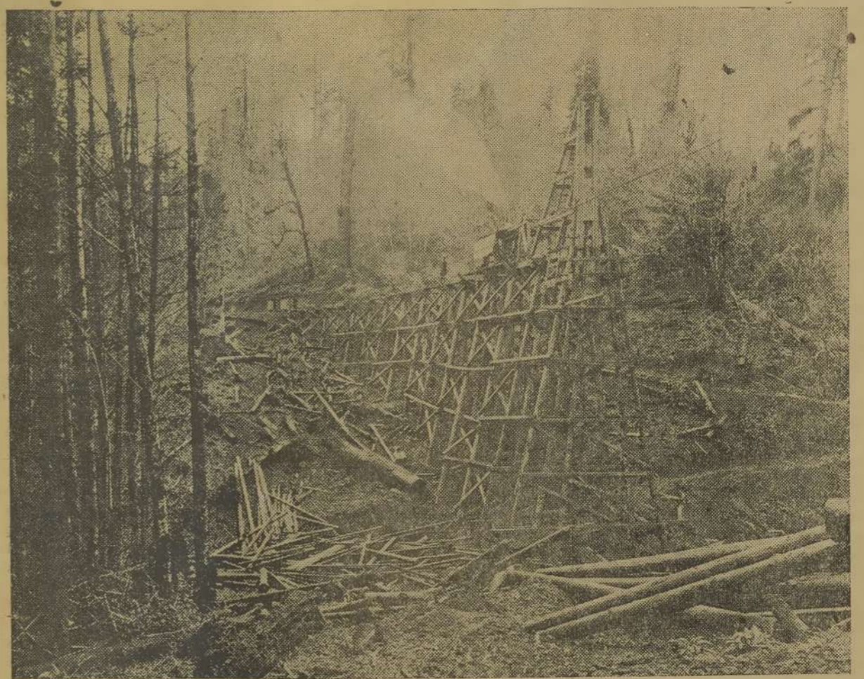
BRIDGE ON GEO. H. CHANEY'S LOGGING ROAD UP GLEN AIKEN CREEK, 600 FEET LONG AND 60 FEET HIGH. THIS ROAD WILL TAP IMMENSE BODIES OF TIMBER.
