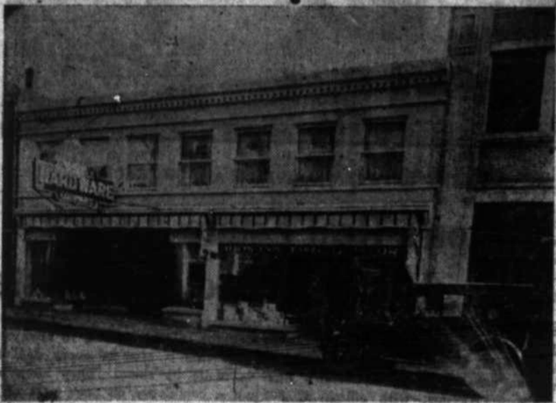
ELLINGSON BUILDING RECENTLY PURCHASED BY COQUILLE HARDWARE CO. OCCUPIED BY THEM AND HUDSON DRUG STORE
