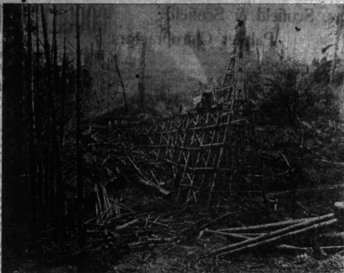
BRIDGE ON GEO. H. CHANEY'S LOGGING ROAD UP GLEN AIKEN CREEK, 600 FEET LONG AND 60 FEET HIGH. THIS ROAD WILL TAP IMMENSE BODIES OF TIMBER.
