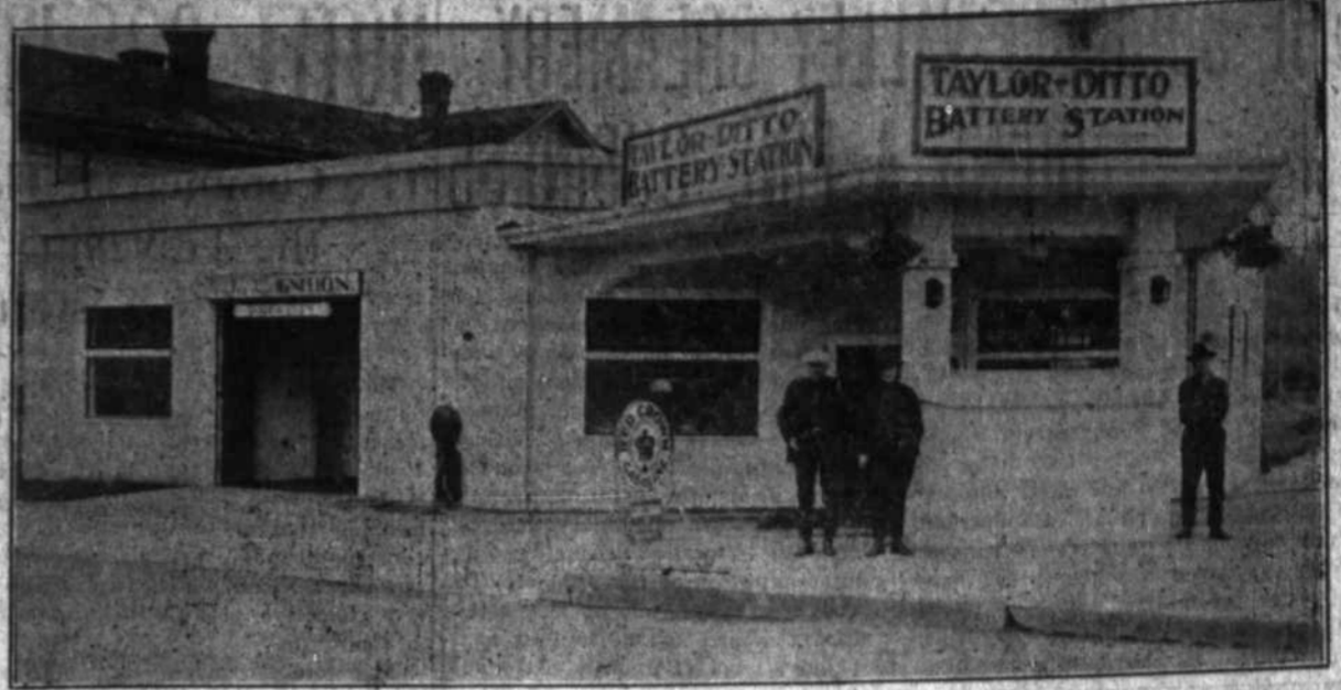
TAYLOR-DITTO BATTERY STATION—ONE OF COQUILLE'S POPULAR SERVICE STATIONS
