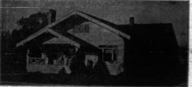
RESIDENCE OF E. E. JOHNSON ON SPURGEON HILL
