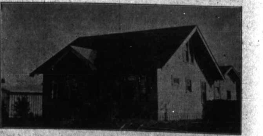
NEW HOME JUST COMPLETED BY W. H. WIMER
