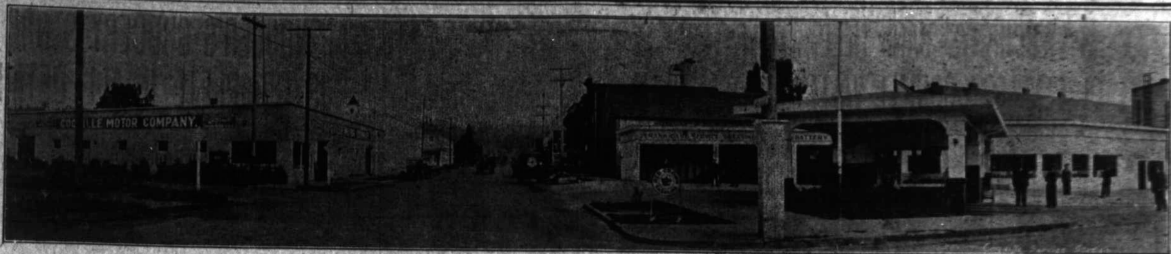
PANORAMIC VIEW OF THE COQUILLE MOTOR CO. GARAGE AND THE COQUILLE SERVICE STATION AT THE CORNER OF TAYLOR STREET, LOOKING UP SECOND.
