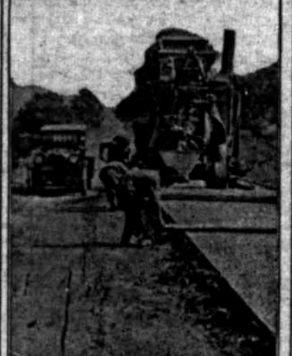
Building on One Side of Road While Other is Open to Traffic.
