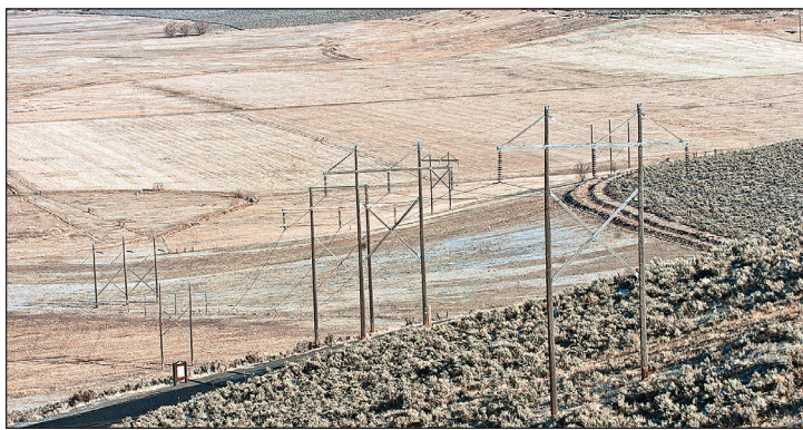
The proposed route of the Boardman to Hemingway power line would replace an existing line just east of Baker City.
