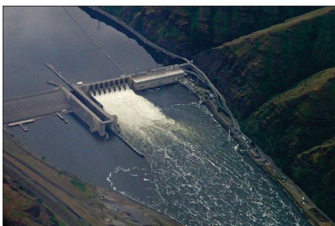
Ted S. Warren/The Associated Press, File The Lower Granite Dam on the Snake River is seen from the air near Colfax, Washington.
