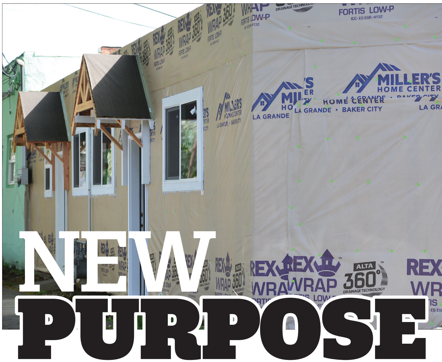
Former chiropractor's office being converted into a lodging site
