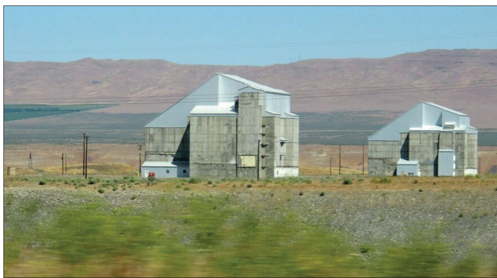
The decommissioned plutonium-producing DR reactor, left, and D reactor, right, are shown on the Hanford Nuclear Reservation, June 13, 2017, near Richland, Washington. The federal government is moving forward with the cost-saving "cocooning" of eight plutonium production reactors at Hanford that will place them in a state of long-term storage for decades to allow radiation inside to dissipate until they can be dismantled and buried.
