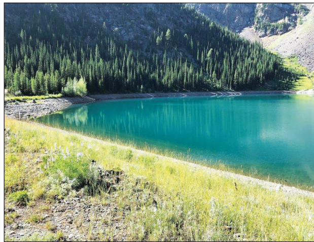
Baker City Public Works/Contributed Photo, File
