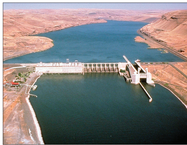
U.S. Army Corps of Engineers/Contributed Photo Washington's Lower Monumental Dam is one of four dams along the Snake River that environmentalists call "salmon-killing machines."
