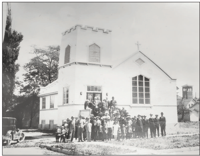
Baker City First Lutheran Church/Contributed Photo
