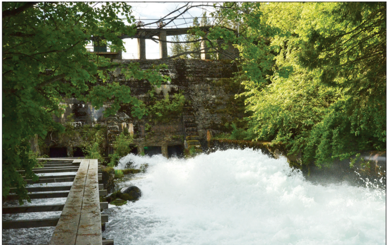
Water from Wallowa Lake flows through the Wallowa Lake Dam at about 400 cubic feet per second early Friday, June 12. The dam is slated for a $16 million refurbishing next year that will include some form of fish passage.
