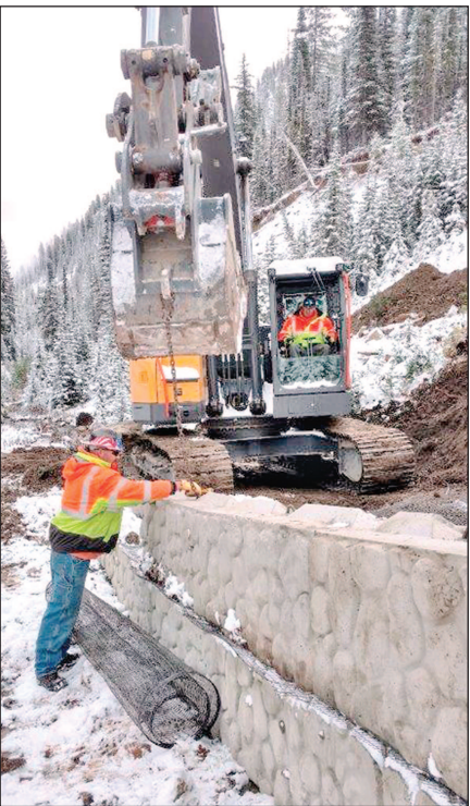
Photo by Tom Fisk, Baker City Public Works Baker City Public Works employees build a retaining wall on a slope that slid in early July. The site is below Goodrich Dam.
