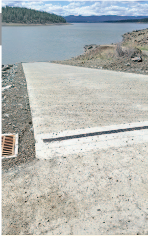
New boat ramp at Phillips Reservoir
