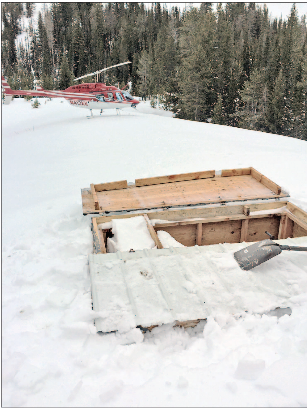
A helicopter ferried Baker City PublicWorks employees to Goodrich Lake on Monday, where they dug out the box that houses a valve controlling water releases from the lake. Goodrich is one of the city's two major supplementary water sources.
