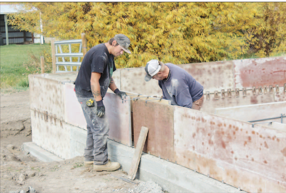
Casey Crowley / Baker City Herald Tyler Shaft, left, and Bodie Barid work on the foundation for one of two duplexes contractor Jeff Petry is building at 10th and Estes streets. Contractor Jeff Petry hopes to finish the two buildings by April 2019.
