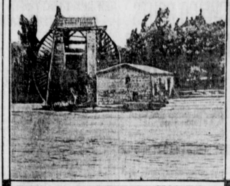
Irrigation Wheel on the Orontes, at Antioch.
