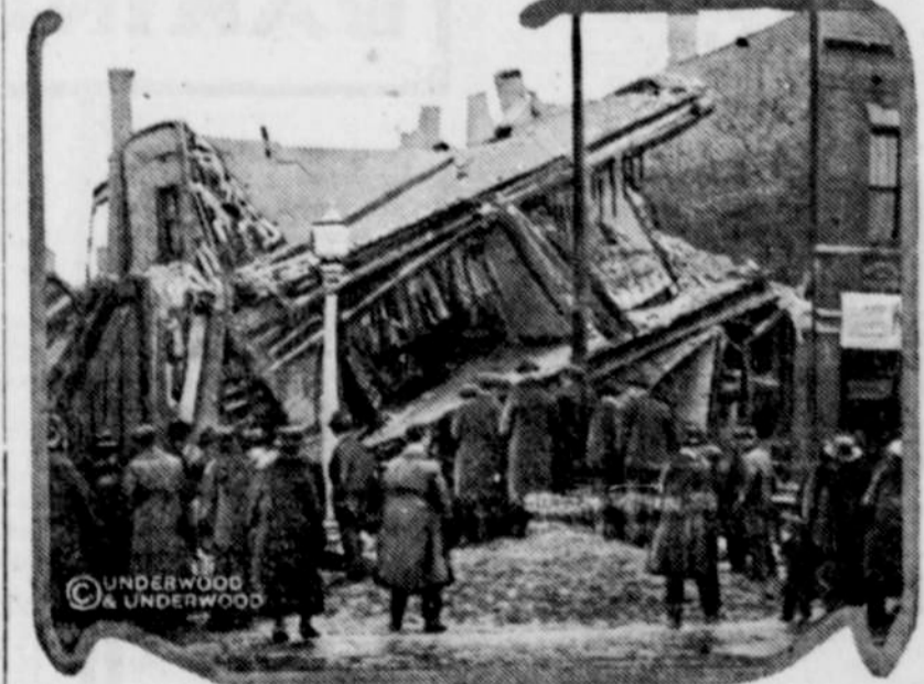
A family of seven fled in panic down a shabby rear stairway on West Madison street, Chicago, and escaped death by a few seconds. As they reached the back yard, the building they had just left collapsed. The building was a two-story brick structure. The rain is believed to have softened the ground beneath the east wall of the building where an excavation had exposed it.
