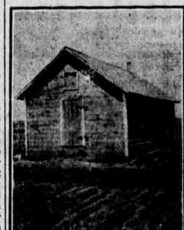
An insulated frame potato storage house used for storing second crop of potatoes at Morrill, Tex.
