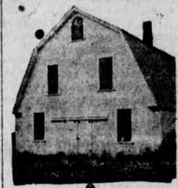
Potato storage house in Maine, showing a central driveway entrance into the lower or basement portion. The end entrance is more commonly used, especially in larger structures, than is the side entrance.
