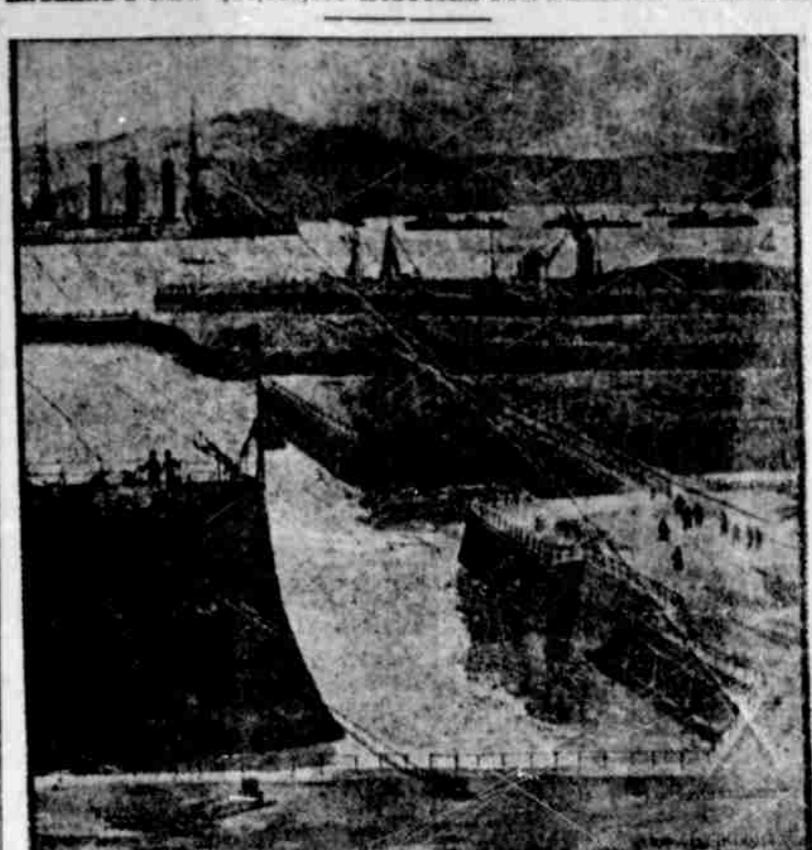
ENTRANCE LOCK TO NEW NAVAL DOCKS AT DEVONPORT. England's new naval works here shown have made Devonport the best equipped and largest war port in the world. They include a fine tidal basin, with an entrance direct from the Humber, and a closed basin, which has been provided with an entrance from the Humber, which can be used for dry docking men of war. Devonport has now three new docks, which can take even the biggest men of war, apart from the entrance lock. It need hardly be pointed out that the final issue of naval warfare depends to a considerable extent on the rapidity with which the opposing nations can refit and replace on the active list battle ships and other war vessels damaged by the enemy. Thus the north extension of the dockyard at Devonport, which was opened by the Prince of Wales recently, must be reckoned among England's most valuable naval assets. The closed basin has an area of thirty-five acres; the extension covers nearly 120 acres. The total cost of the new work was about $4,500,000.
