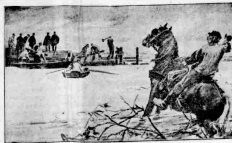
HOLLANDERS WORKING TO FILL UP CRACK IN DIKE NEAR HORN.
