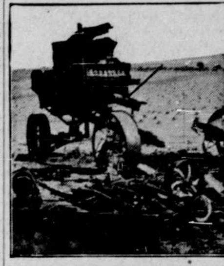
Thrashing Outfit Destroyed by Grain Dust Explosion.
