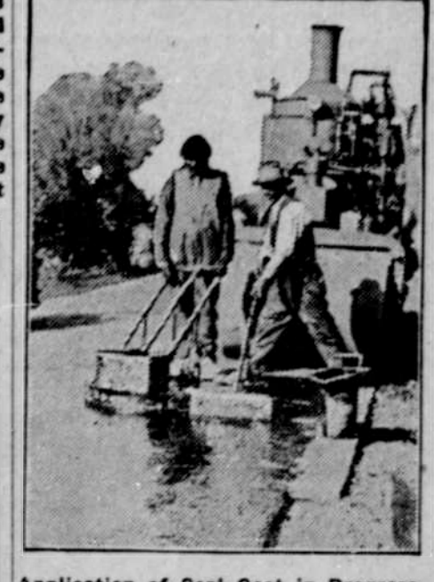
Application of Seal Coat in Progress.
