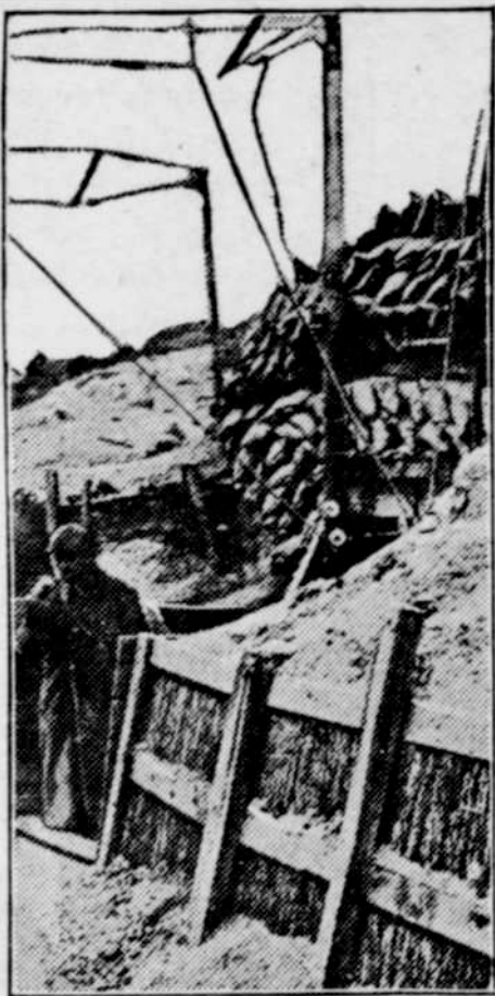
Entrance to a Dugout.
