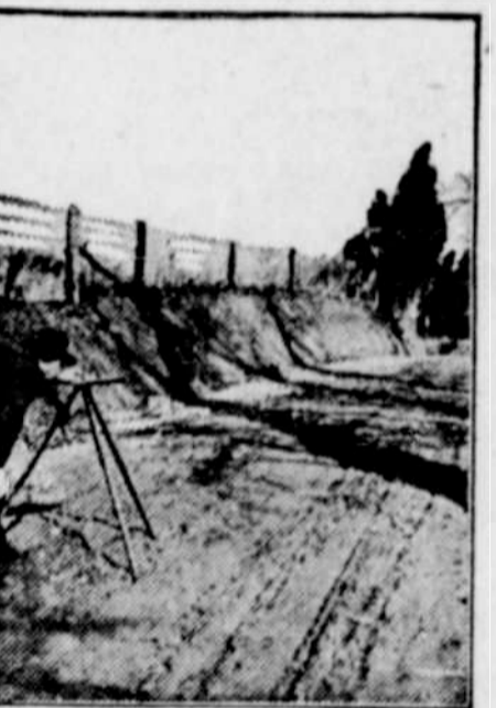
Getting Road Levels Preparatory to Improving Highways.
