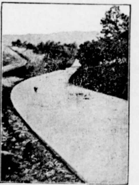
Concrete Road in Suburbs of Chicago.
