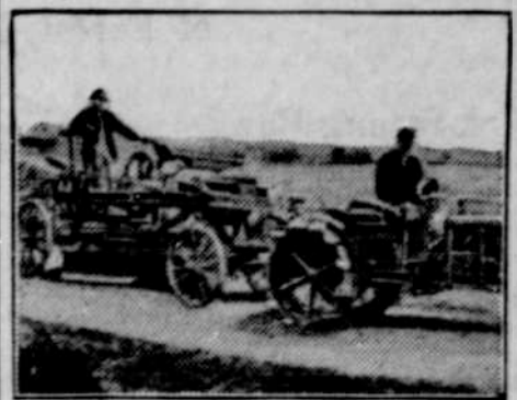
Efficient Aid in Road Repairing.
