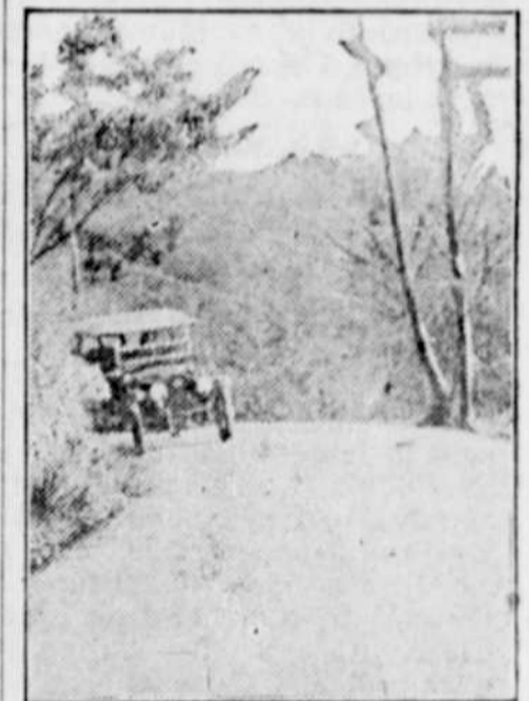
Superior Type of Concrete Road.
