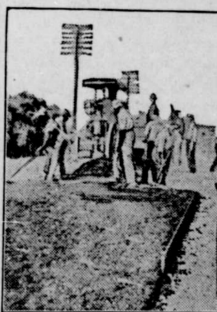
Building Asphalt Pavement.
