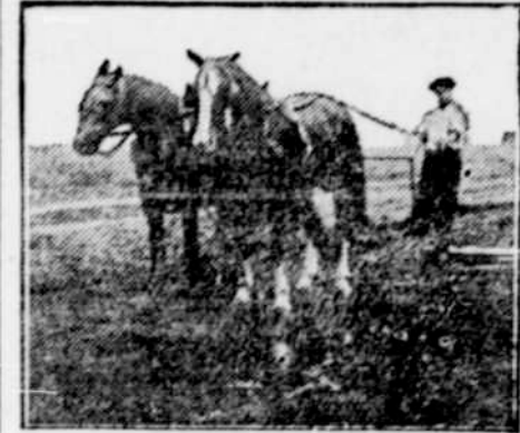
Operating a Road Drag.
