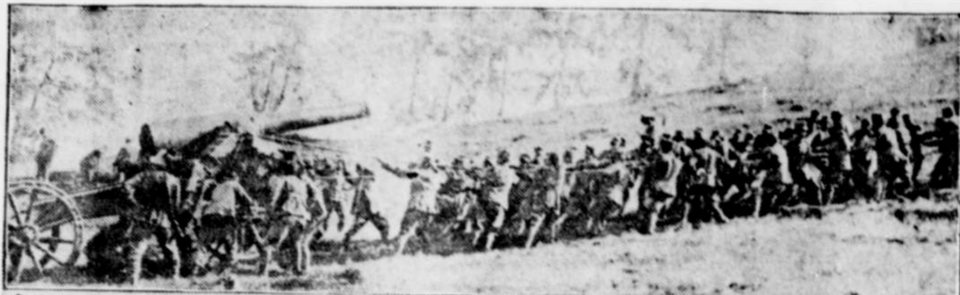
PULLING BIG ITALIAN GUN INTO POSITION UP MOUNTAIN
