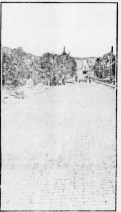
CONSTRUCTING A BRICK ROAD.
