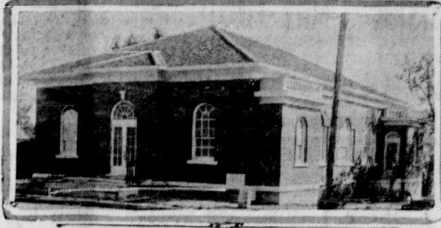
First Church of Christ, Scientist, now nearing completion, Corner A Street and Pacific Avenue. Photo by Bryant)
