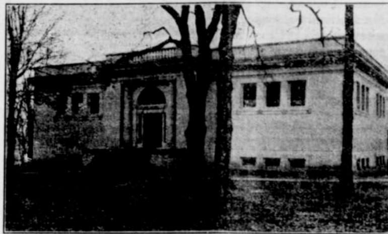
THE NEW CARNEGIE LIBRARY OF PACIFIC UNIVERSITY FROM THE NORTH
