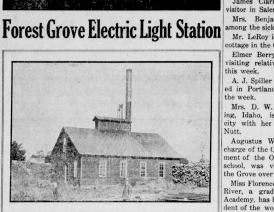
This wooden barn covers ONE boiler, ONE engine and ONE generator [or Dynamo] which constitutes the entire mechanical installation which provides electric light during NIGHT HOURS in the GROVE. IF ANY PART OF THIS PLANT BREAKS DOWN the entire service is interrupted. If you
