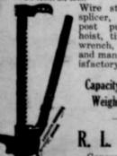
Wire stretcher and splicer, lifting jack, post puller, press, hoist, tire tightener, wrench, vise, clamp, and many other sat-isfactory uses.
