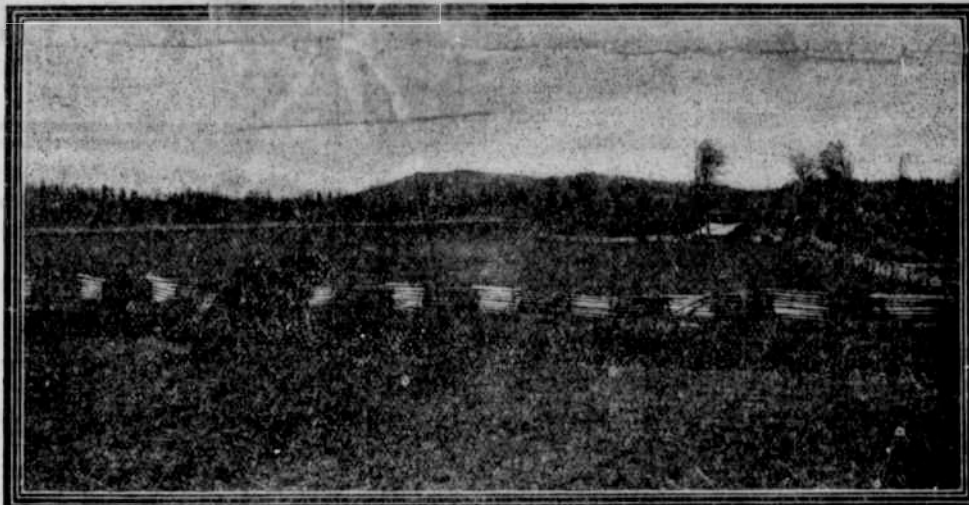
GETTING READY THE GROUND.
