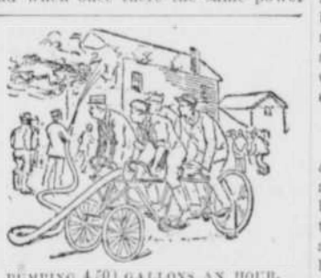
PUMPING 450 GALLONS AN HOUR.
