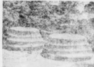
Typical 80-ton Bakelite plastic silos.
