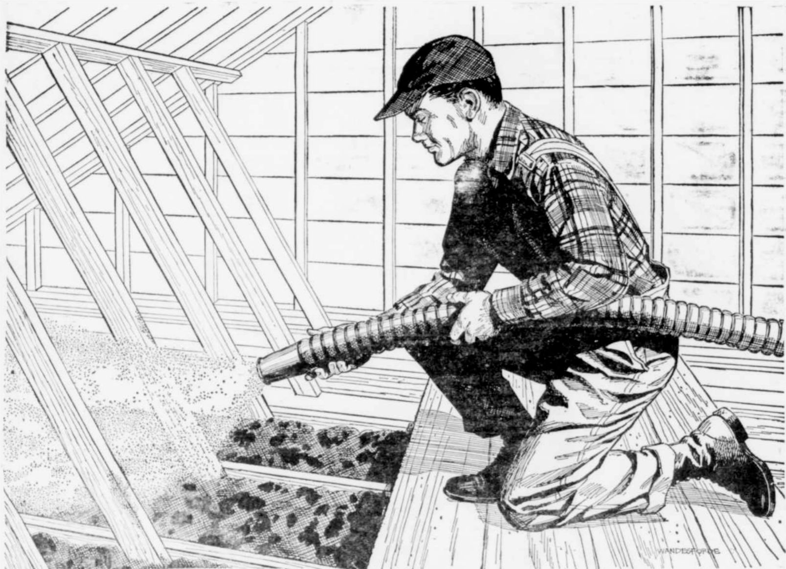
Silvawool—scientifically processed wood fibers—is an efficient insulation. Professionally applied, the "blown-in" method fills every corner and crevice, forming the insulation into a fluffy mat that locks out heat or cold. In the manufacturing process the wood fibers are impregnated with fire and moisture retardants. For homes, refrigerated warehouses or food locker plants, Silvawool helps maintain steady temperatures, with minimum fuel and power cost.
