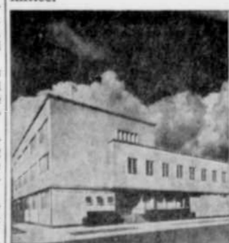
Headquarters of the National Congress of Parents and Teachers stands today at 700 North Rush Street, in Chicago. The building, dedicated in 1955, won an award from the Chicago chapter of the American Institute of Architects and the Chicago Association of Commerce and Industry for excellence in architecture.
