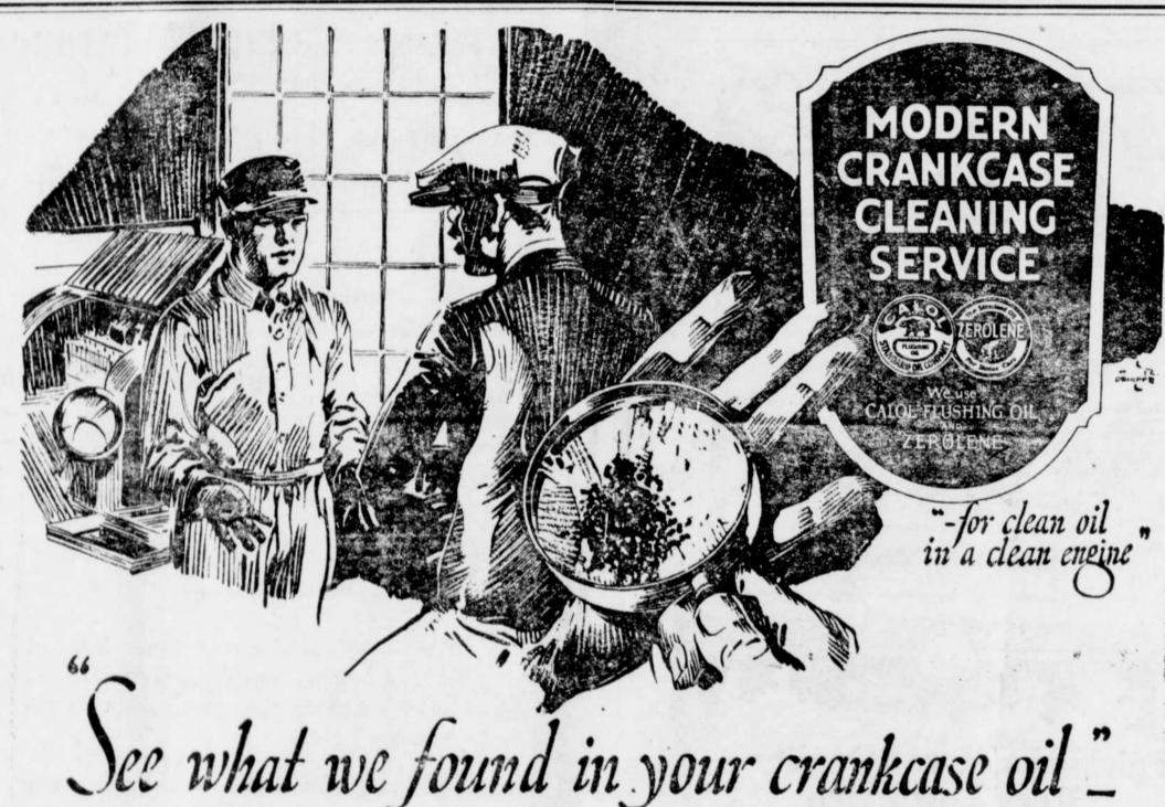
THIS lens shows some of the dirt that can be found in any crankcase after a few weeks of driving—road dust, carbon and fine particles of metal. Such dirt circulates with the lubricating oil through the engine, together with gasoline that cscapes past the pistons and dilutes the oil.
