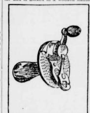
Pivoted to the center is a revolving handle resembling a miniature motor man's controller, with a little cup in one end to hold the kernel and a spring cap to keep it in place and press it against the grater plate. The nutmeg is placed in this cap and the handle turned until the desired amount to be thrown away.
